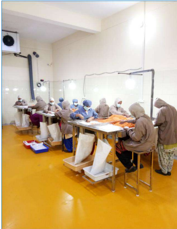
PU Flooring in Packing Room
